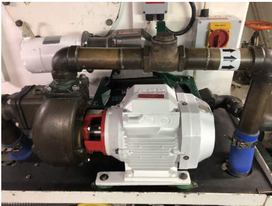
Fire / bilge pump serviced and painted
